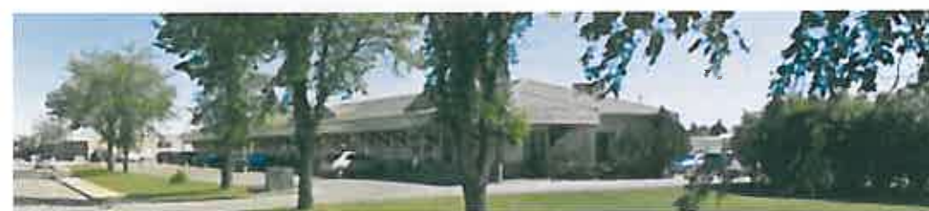
(Photo to Left) An example of a building on a narrow strip of land along railway.
