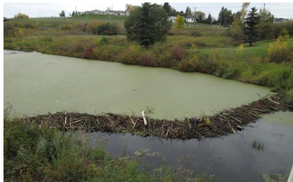
Photo: Beaver dam south of pedestrian bridge
